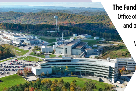
The Spallation Neutron Source produces neutrons with an accelerator-based system that delivers microsecond proton pulses to a steel target filled with liquid mercury through a process called spallation. The neutrons are directed toward state-of-the-art instruments that provide a variety of capabilities to researchers across a broad range of disciplines including physics. Credit: ORNL, U.S. Dept. of Energy
