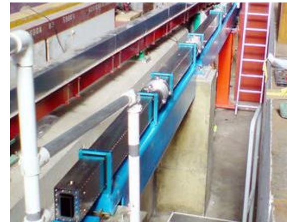
Guide Installation at ISIS
